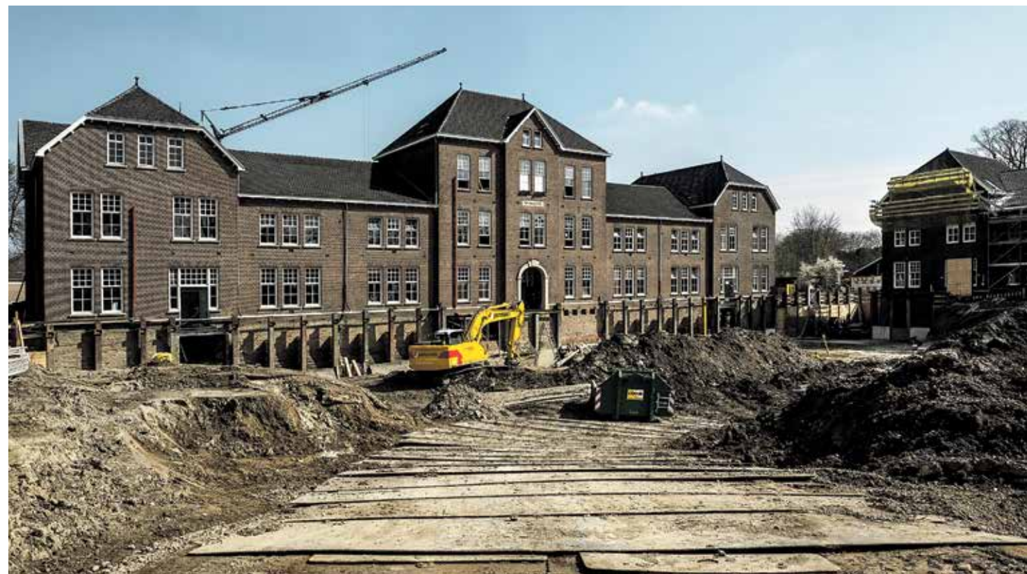
Tapijn under construction Photo: Joey Roberts
